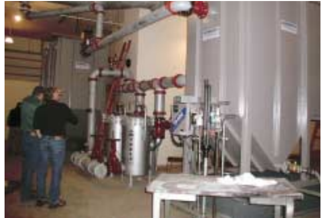
U.S. Army Corps Dam inspection.
