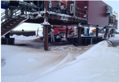
Portable containment placed under the release point to prevent further tundra impacts.
