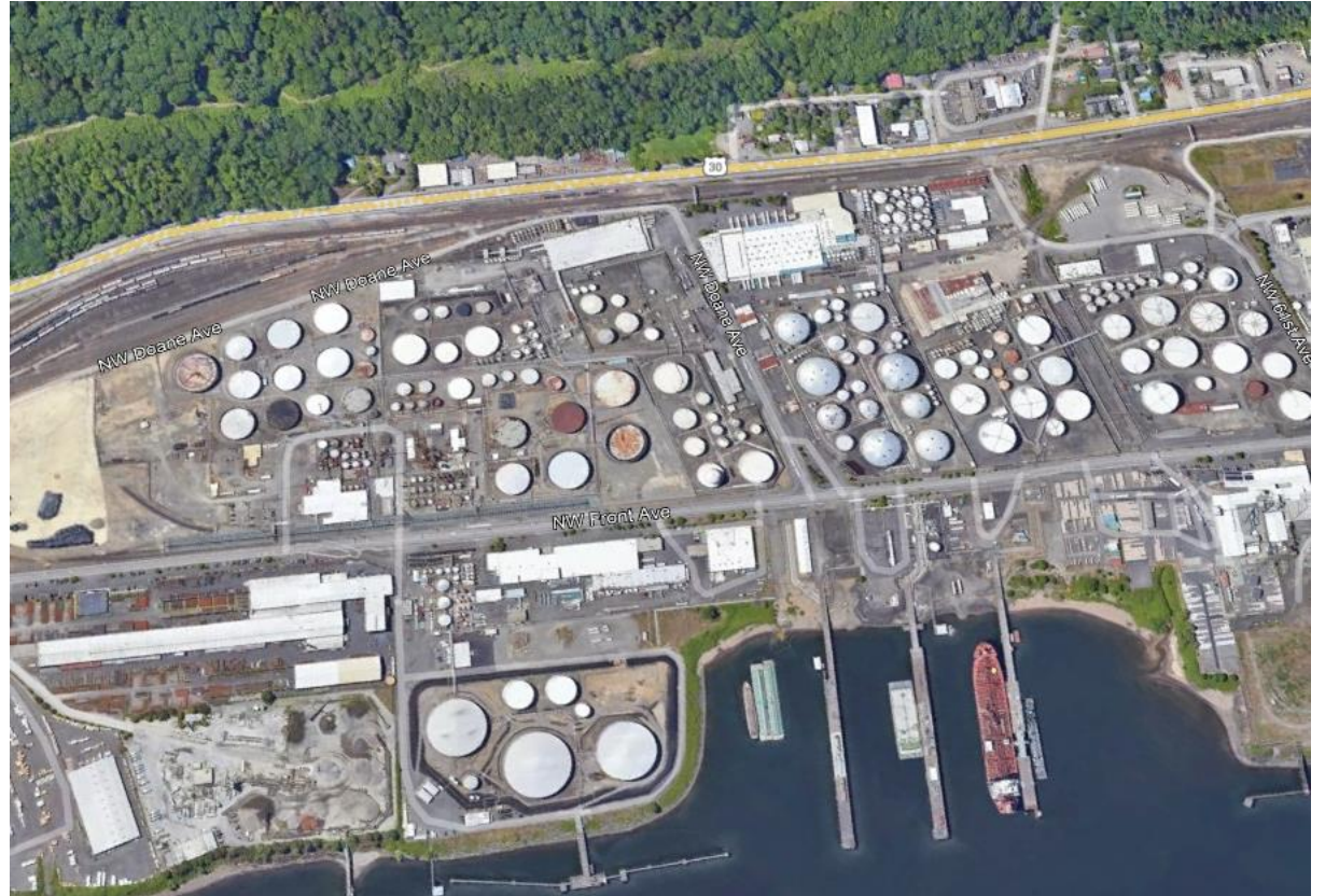
Portland's Critical Energy Infrastructure (CEI) Hub
